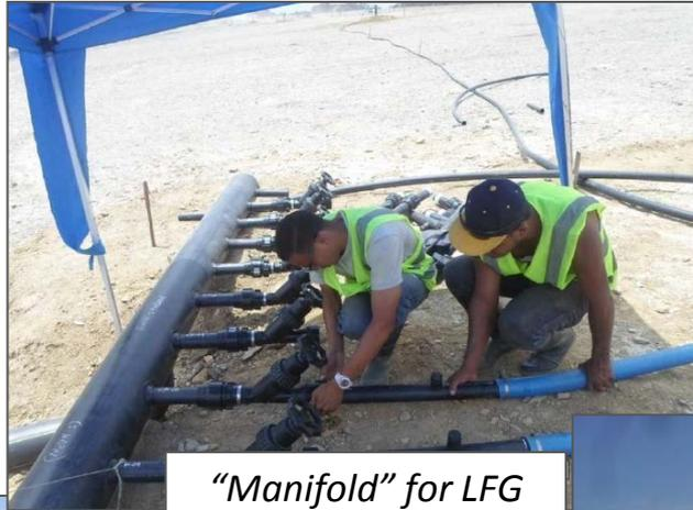
*"Manifold" for LFG active flaring regulation*
