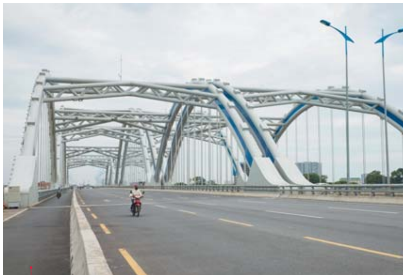
Hanoi, Vietnam - Aug 30, 2015; The Dong Tru arch bridge, made of steel tubes filled with cement, was opened for safety testing in Hanoi on October 2014 as part of the extended Highway No. 5 project. Hanoi / Shutterstock.com
