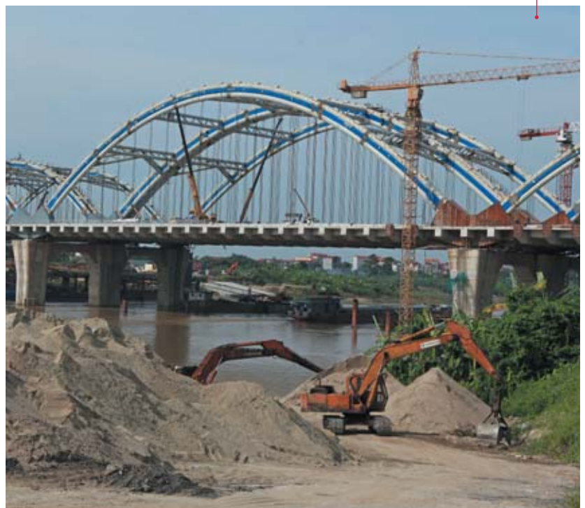
HANOI, VIETNAM - SEP 7, 2014: An under-construction bridge connecting the two parts of Red river in Hanoi capital. Asia Images / Shutterstock.com
