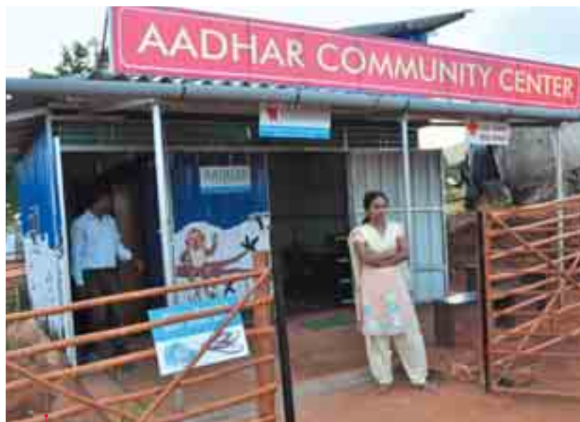
Integrated Energy Centre in Kanbargi with Mahesh Foundation serves as a solar powered community centre with education and health facilities, in addition to being a charging station for lights and mobile phones - Source: SELCO Foundation
