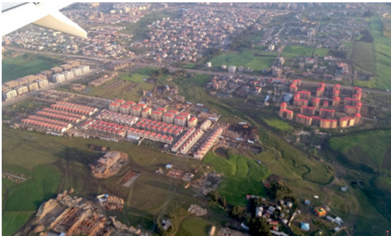
Condominium housing development in the eastern part of Addis Ababa, Ayat area - ©Hany Abo El Wafa
